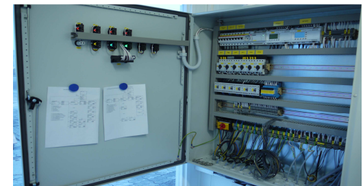
control cabinet separate or on DAF reactor
