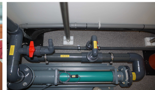
feeding / standard ISO container installation 10.0m 3 /h , 30%Recycling, 220 m 3 /day
