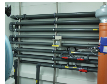
saturation, mixing, aeration polymer prepare station
