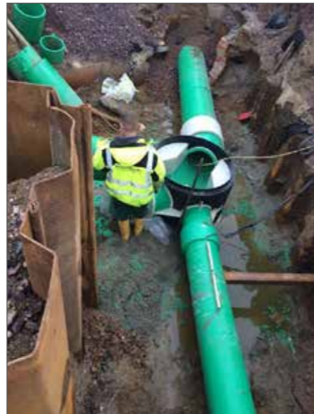
Sewer renovation – PP chamber and PP pipe welded
