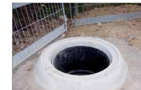
11.) Restoring of road construction incl. decoupled load cover
