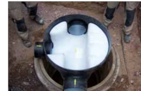
4.) Adapt the prefabricated channel with PE socket
