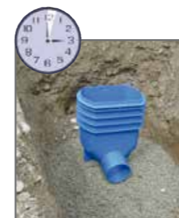
3. Min.: bedding in lean concrete mix
