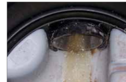
7.) After the filling mortar has hardened, water retention can be removed
