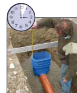
5. Min.: height adjustment
