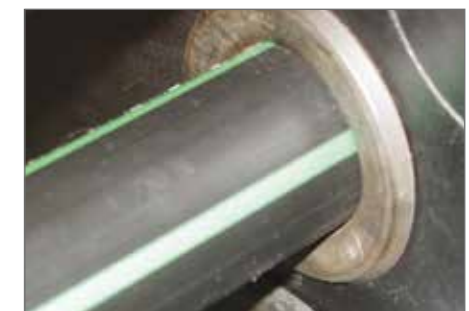
Pipe connection with seal watertight to 0.5 bar
