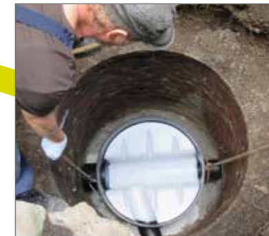
Lower new base into the chamber
