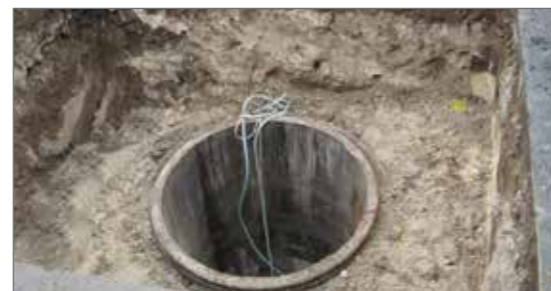
1.) Cut the asphalt, and lift the concrete cone
