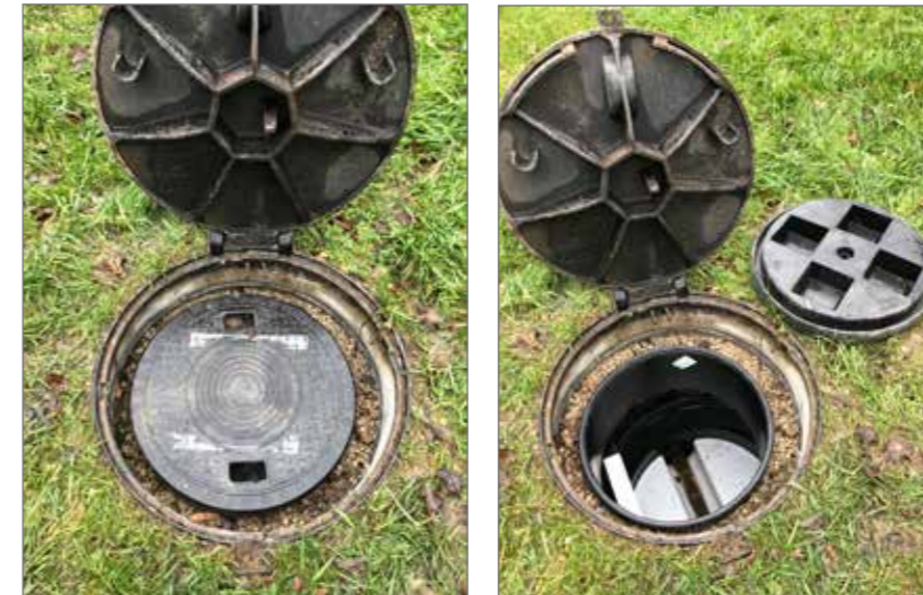
Cover-in-cover solution: Sealing function by PE cover DN 625 Bearing function with standard cover DN 800, class D 400
