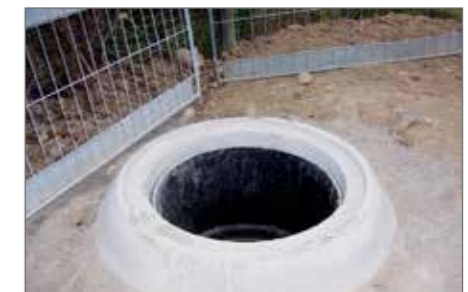
10.) Filling the gap. Restoring of road construction incl. decoupled load cover
