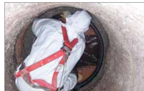
6.) Fitting the ROMOLD element seal on the mounting ring. 100 % watertight transition to the manhole..
