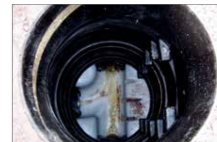
10.) Renovated manhole. Steps were removed on customer request
