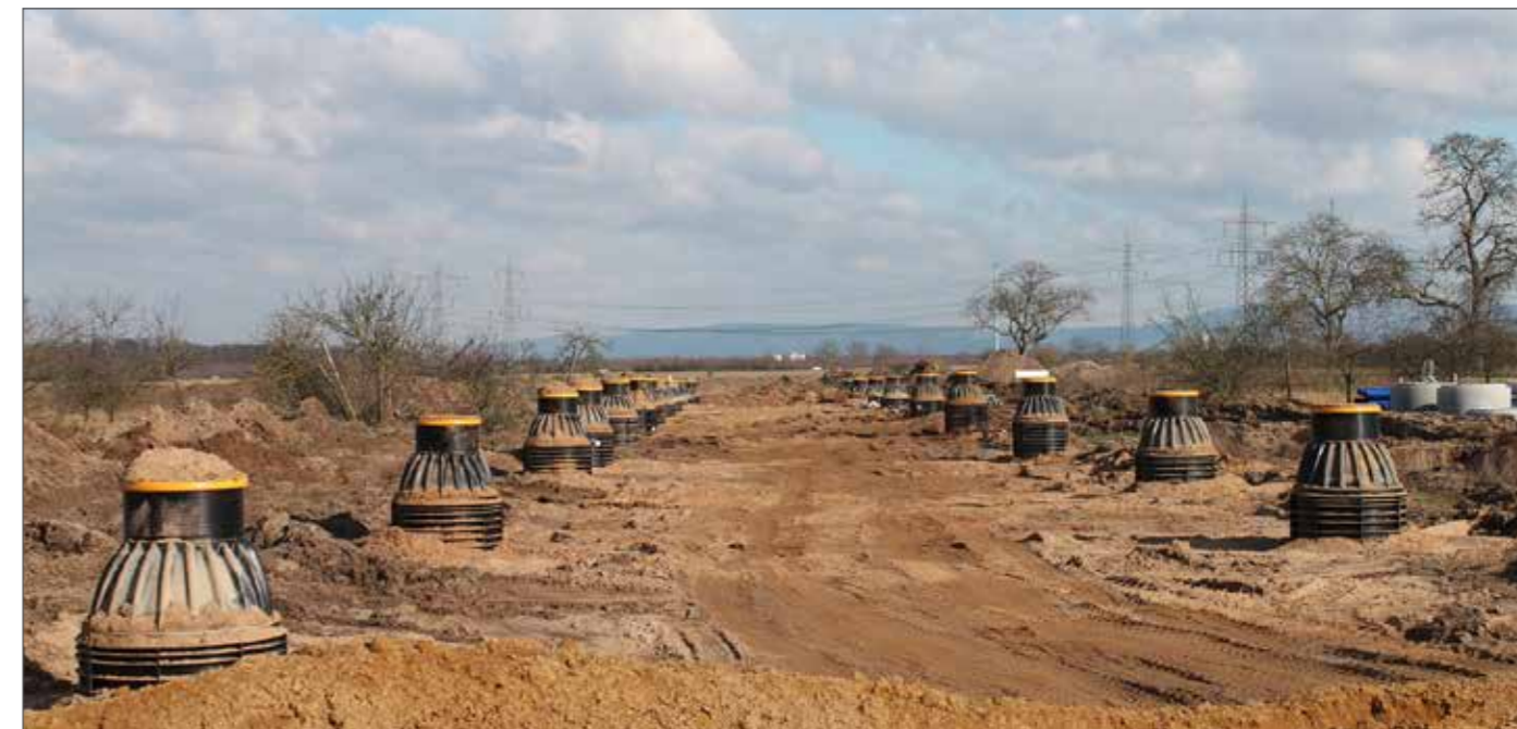
housing development / PP domestic connection chambers DN 1000
