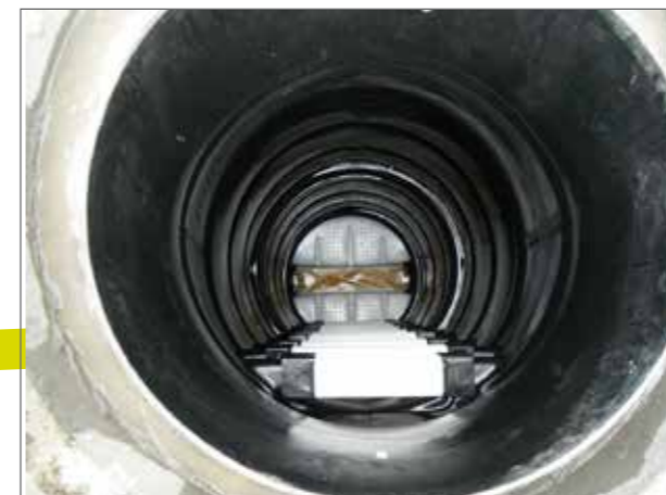
New PE chamber DN 800 in corroded chamber DN 1000
