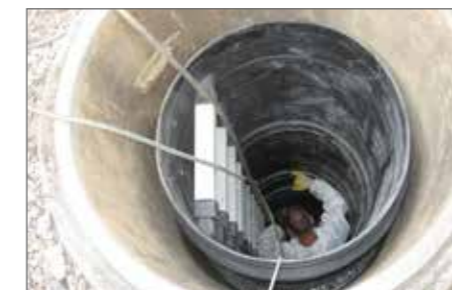
8.) Fitting the seals and chamber components - PE shaft system DN 800
