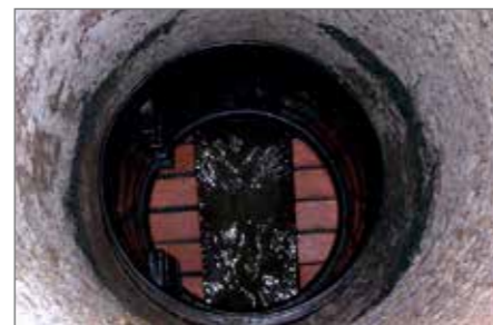
8.) Fitting the seals and chamber components - PE chamber system DN 800
