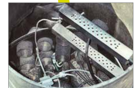
Climbing steps can be easily removed if necessary (cable installation).
