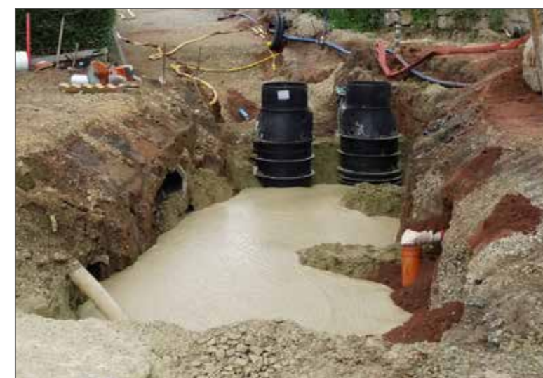
Chamber in controlled low strength material (flowable fill)
