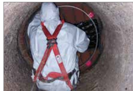
4.) Fix the mounting ring on the berm
