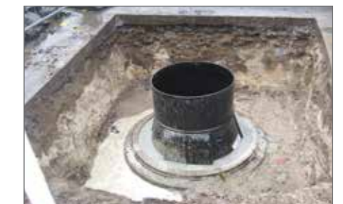
9.) Filling the gap between DN 800 PE chamber and DN 1000 concrete manhole with filling mortar
