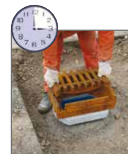
15. Min.: assembly of grating
