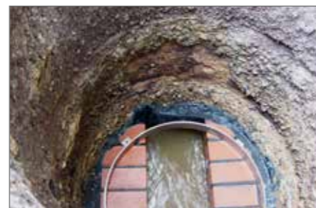
5.) The picture shows the fixed mounting ring
