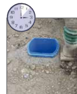
7. Min.: backfilling and compacting
