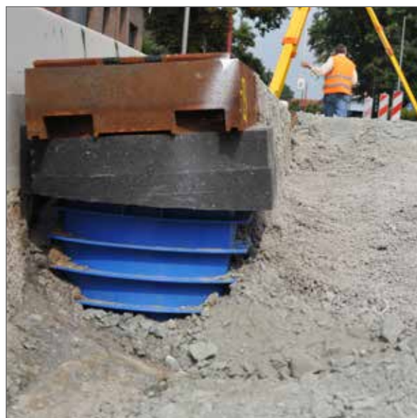
Bearing rin in v-shaped version
