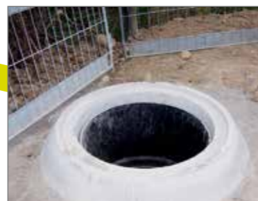
Load decoupled cover
