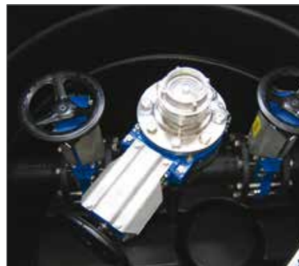
Flushing Manhole DN 1000 3 Slide Valve
