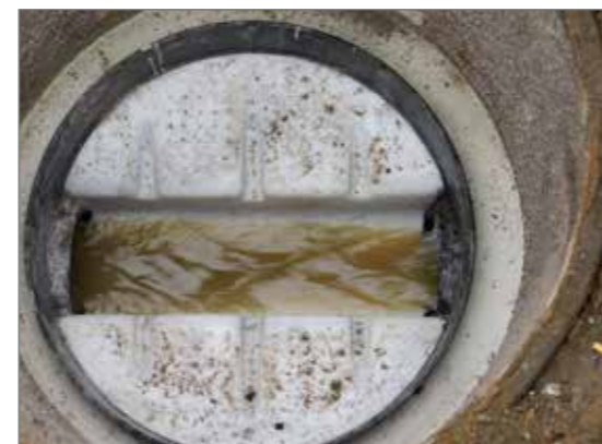
Shaft-in-shaft renovation
