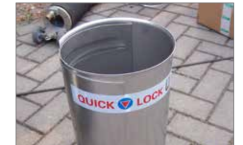
The PE pipe is connected to the old pipe either using Quicklock collar or with construction chemicals
